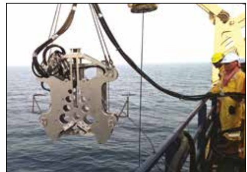
▲ MDWS Diamond Wire Saw lowered into sea.
